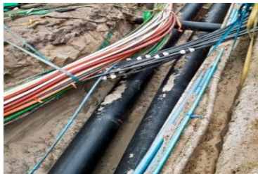
Lay Fiber Optic Cable
